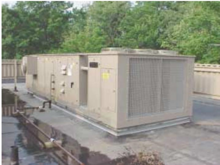
Nesbitt pioneered the development of the rooftop multizone system to accommodate the thermal requirements of multiple learning spaces. In addition to meeting the demands of educators for divisible learning spaces, the rooftop multizone systems helped to reduce the cost of construction in a period of escalating prices. The entire heating, ventilating and air conditioning
