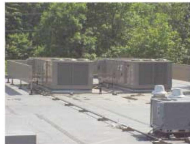
curbs, electric power and gas lines were reconnected and all ducts and control wiring reinstalled. All systems were operational before anyone returned to the building on Monday morning. The building owner / operator suffered no downtime and the savings achieved from the standpoint of actual costs were substantial.
