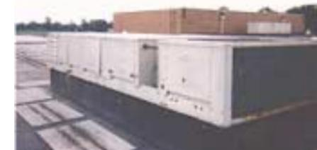
Modification of existing duct connections and control zones can get expensive. The replacement unit that duplicates the original number and size of ducts and control zones can simplify the task and save time and labor.
